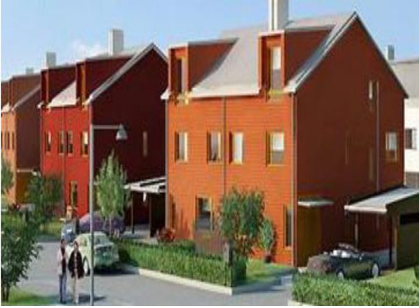
Fig. 2. Some of the semi-detached houses in Stockholm that were selected for study.
